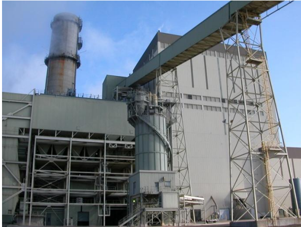
FIGURE 7: A VIEW OF THE MAIN CONVEYOR AS IT HEADS INTO THE POWER PLANT BUILDING. THE TOP OF THE BUILDING IS ABOUT 13 STORIES HIGH.
