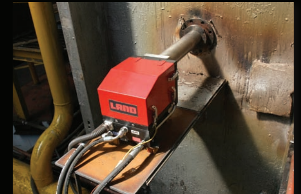
Typical installation showing the FTI-Eb mounted into a process - the sensor is shown in the protective enclosure
